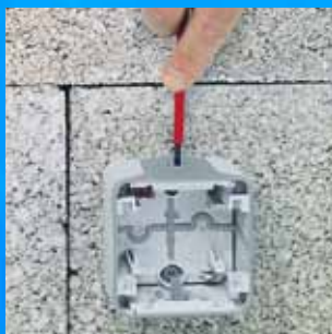
1/ Pierce the end cap using a screwdriver
