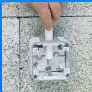
2/ Insert the tube through the end cap
