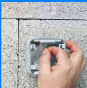
1/ Make the end cap cut-out by pulling the seal
